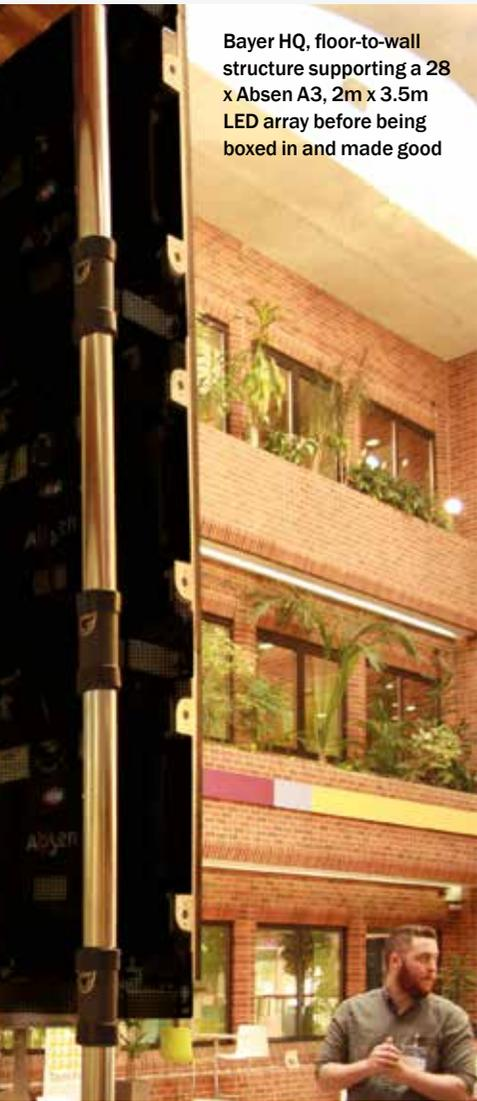
Bayer HQ, floor-to-wall structure supporting a 28 x Absen A3, 2m x 3.5m LED array before being boxed in and made good
